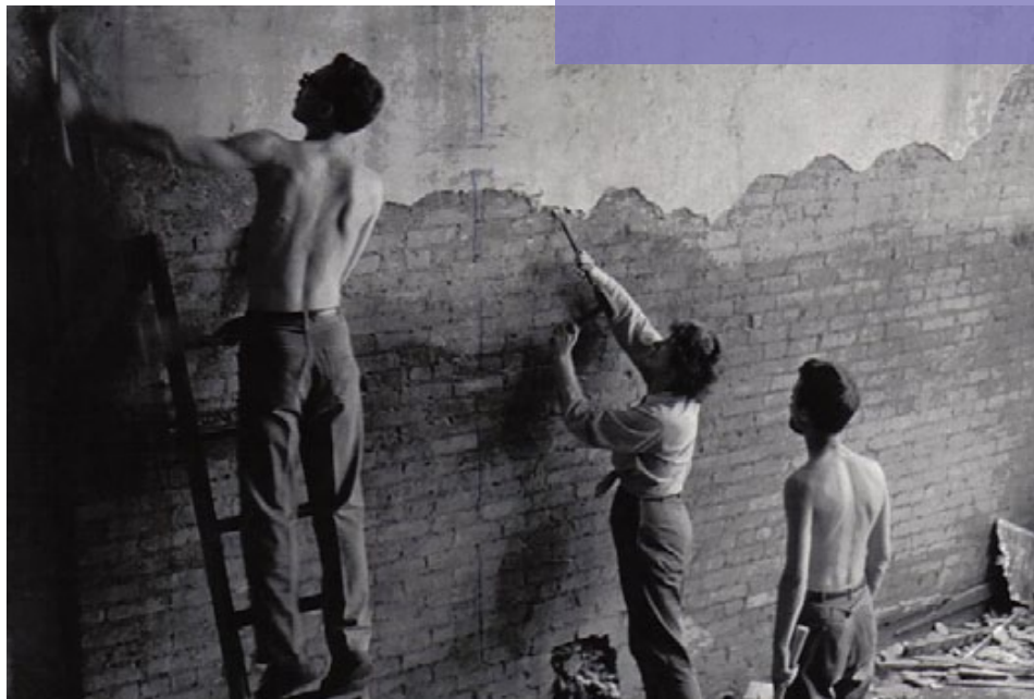
Residents exposing a brick wall in a loft on Broome Street, 1974 (Photo from Dorothy Koppelman)
